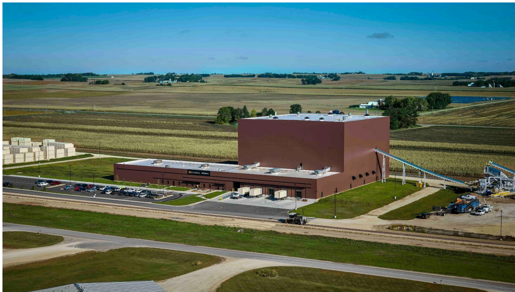
Front elevation of new Cambria Quartz Processing Center in Randolph, MN
